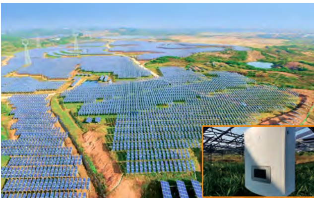
Zhejiang Hangbu Agricultural-photovoltaic hybrid PV plant 30MW
